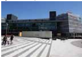
Spain PTA Malaga
